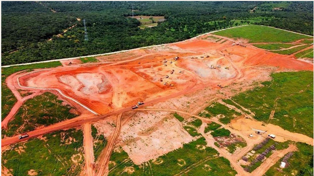
Construction of Sigma Mineração's lithium concentrate production and processing plant.
