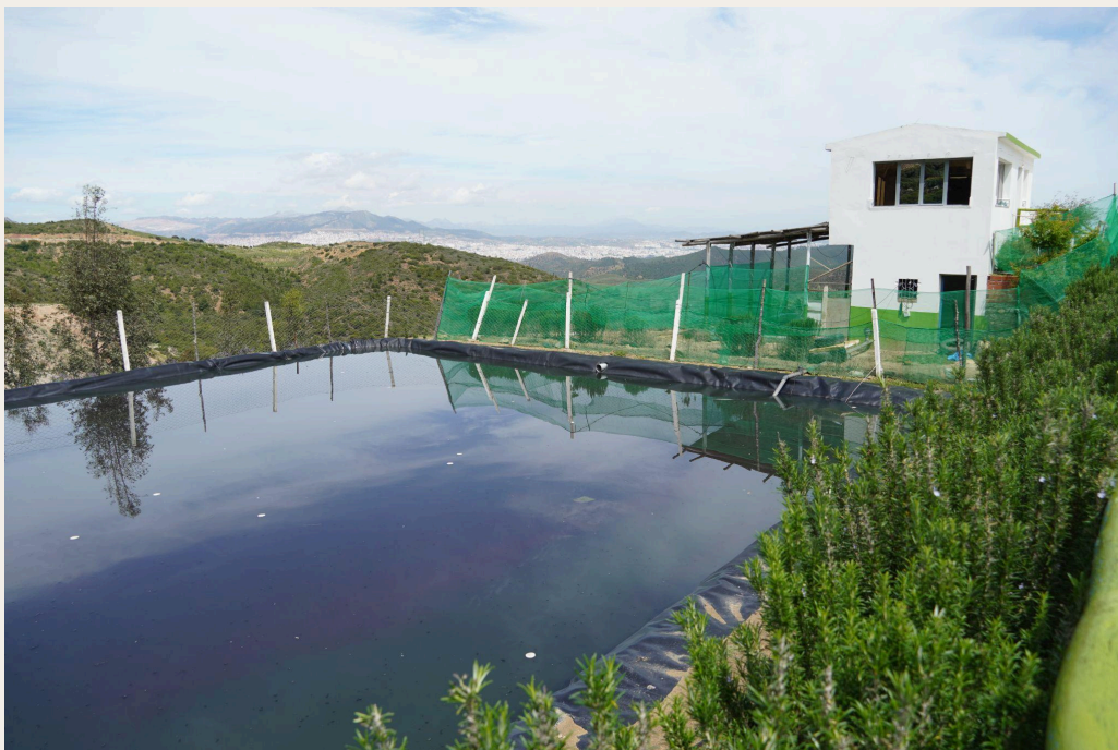
Water Storage Tank and the Storage Pond. Photo: Xiao Chenjuan.
