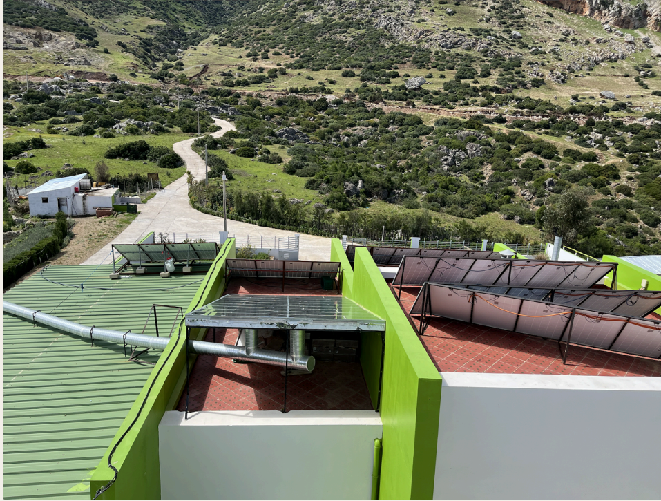
Solar Panel and Air Source Heat Pump. Photo: Xiao Chenjuan.
