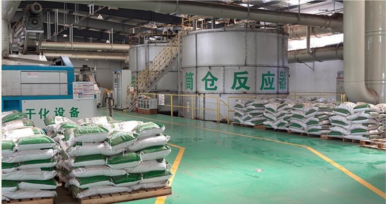
Demonstration Center for the Treatment and Use of Urban and Rural Organic Waste in Linhu, in the city of Suzhou - Mauro Ramos
