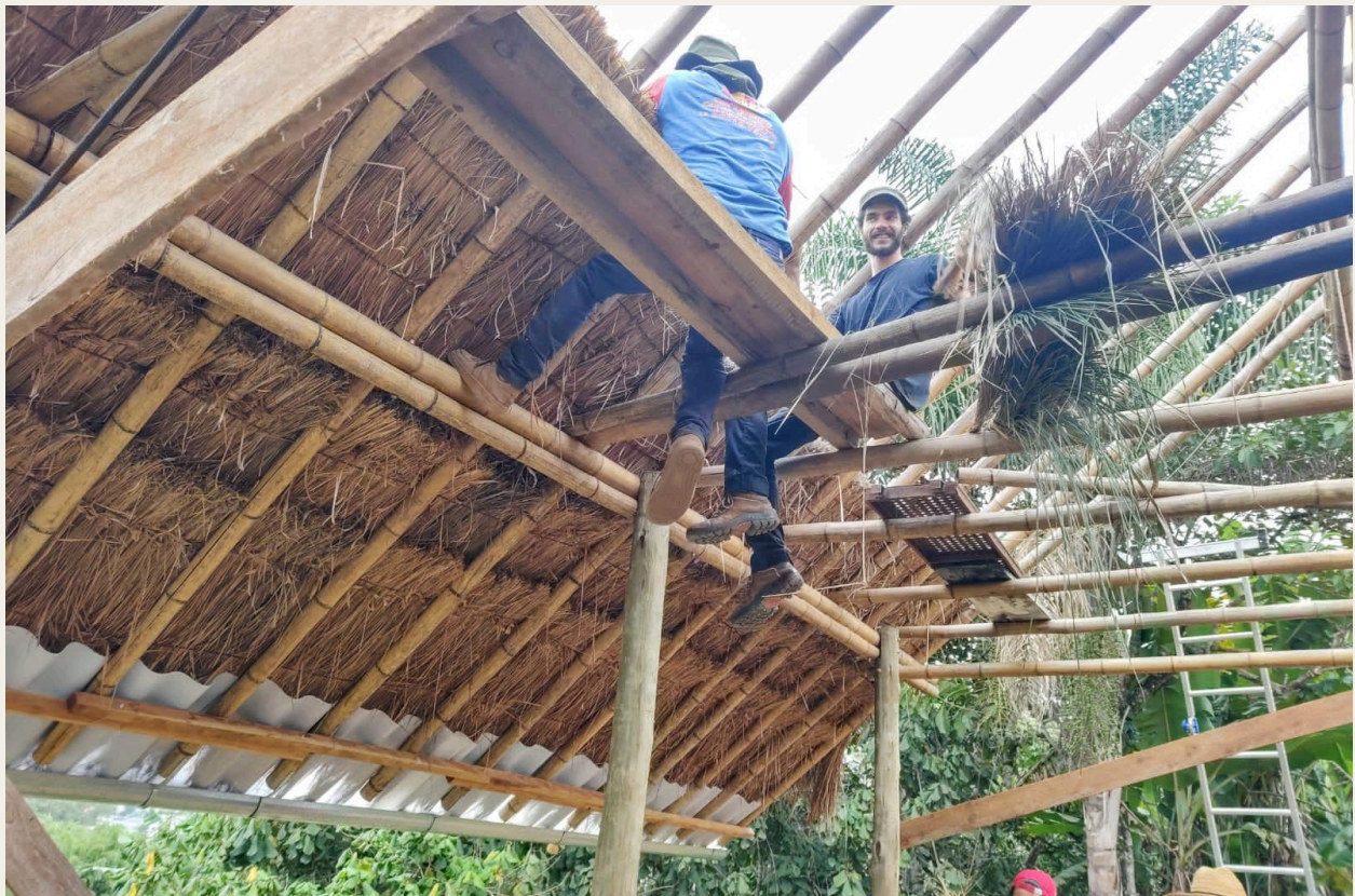
Construction of a bamboo and straw roof. Photo: MST-SP and FAUUSP archives.
